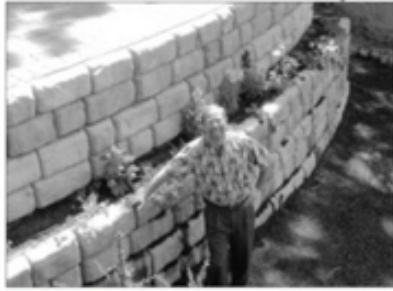
And Now Dan Houk stands proudly in front of a wall of Red-Block recently completed for a residence.
